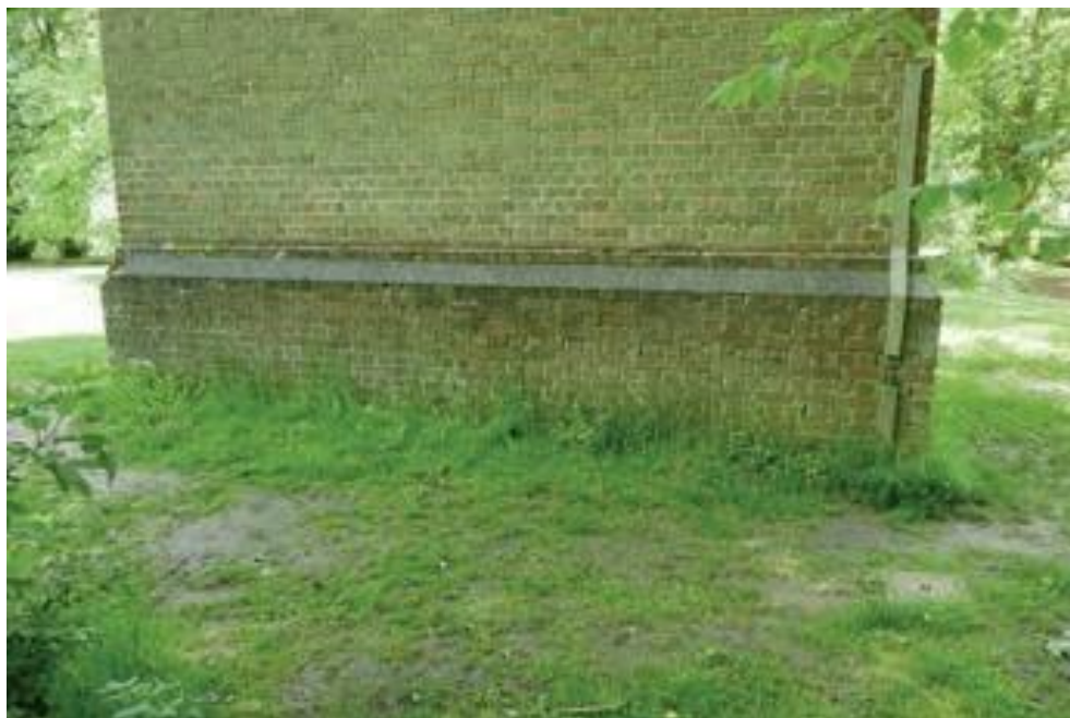
Figure 7 General view of plinth
