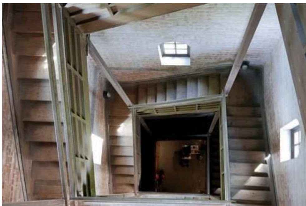
Figure 22 General view of stair
