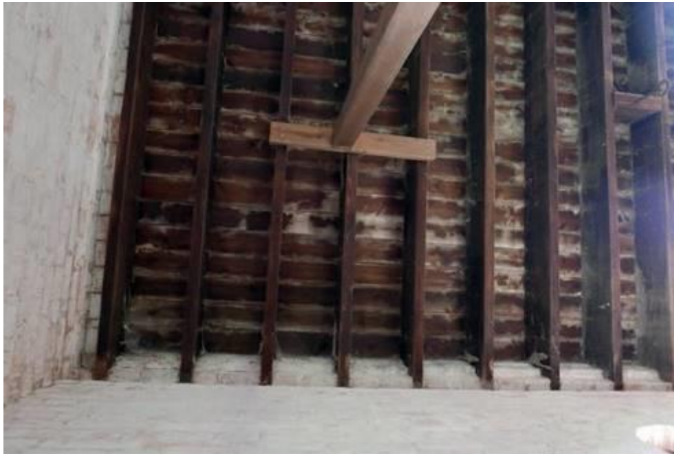
Figure 21 General view of Belvedere floor structure
